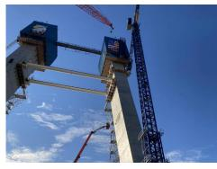
A walkway connecting the jump forms on the north and south tower legs has been installed on the Canadian and US sites. Currently sitting approximately 40 metres/120 feet above the ground, it gives workers access to and from each tower leg during construction. As the jump forms rise, so too will the walkway.
