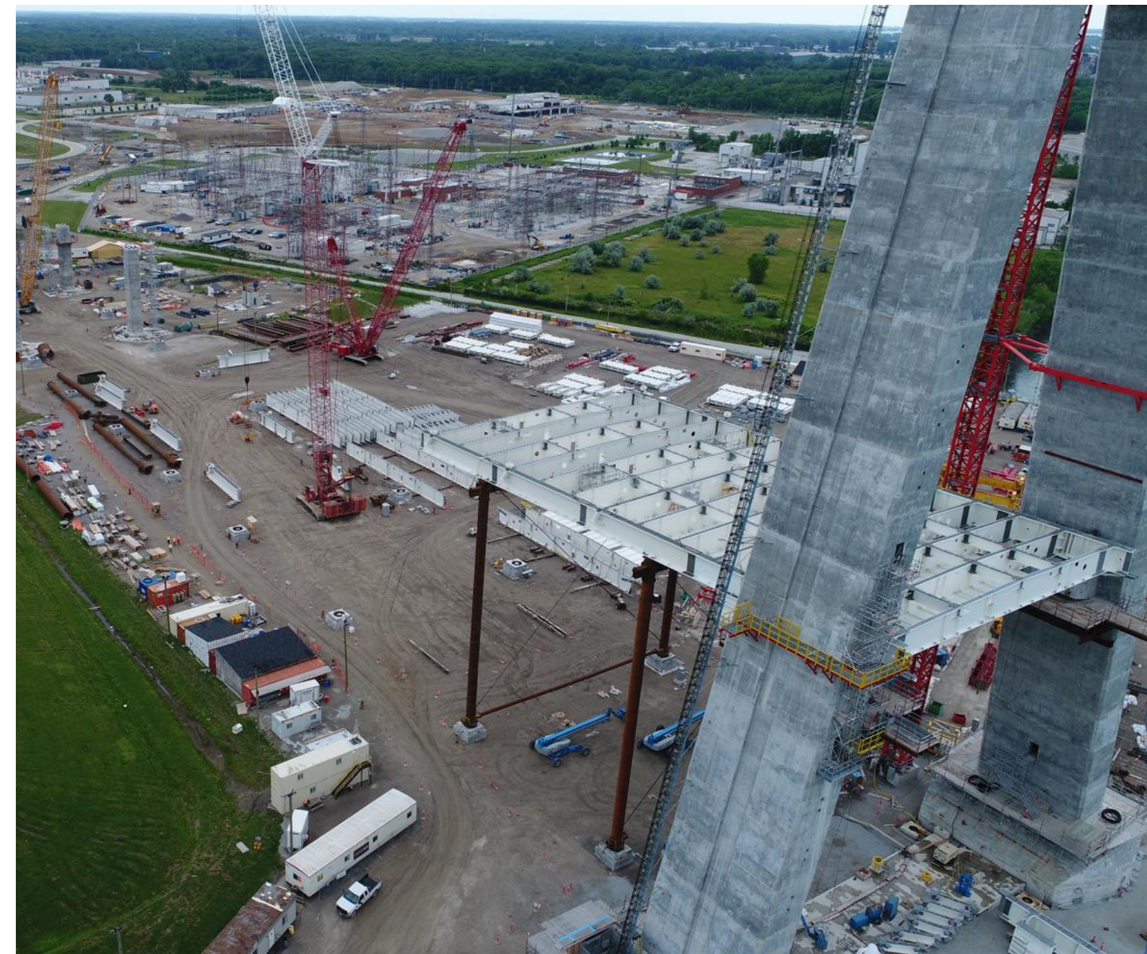
Canadian bridge site: tower and side span work
