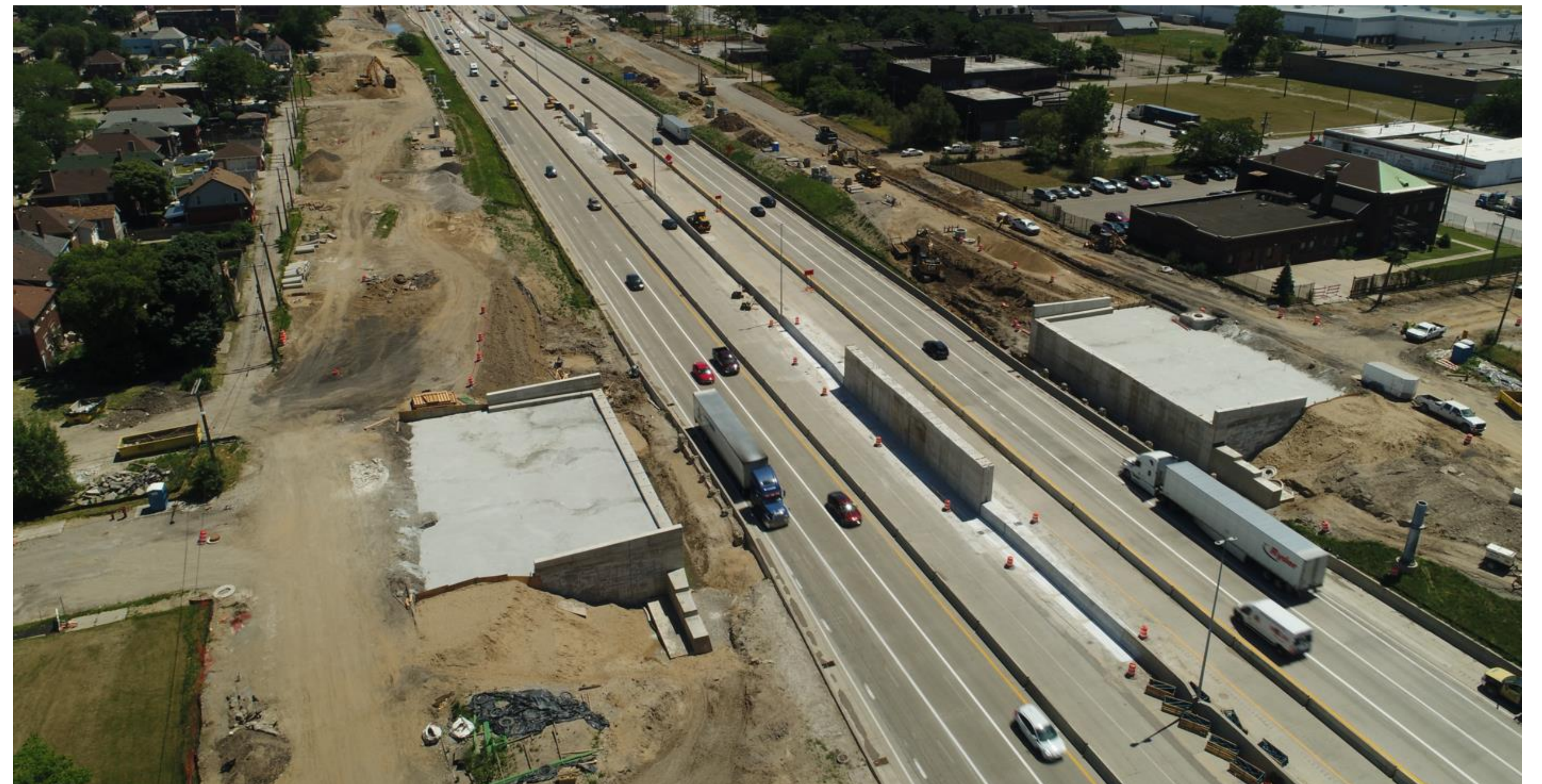
Green Street road bridge construction
