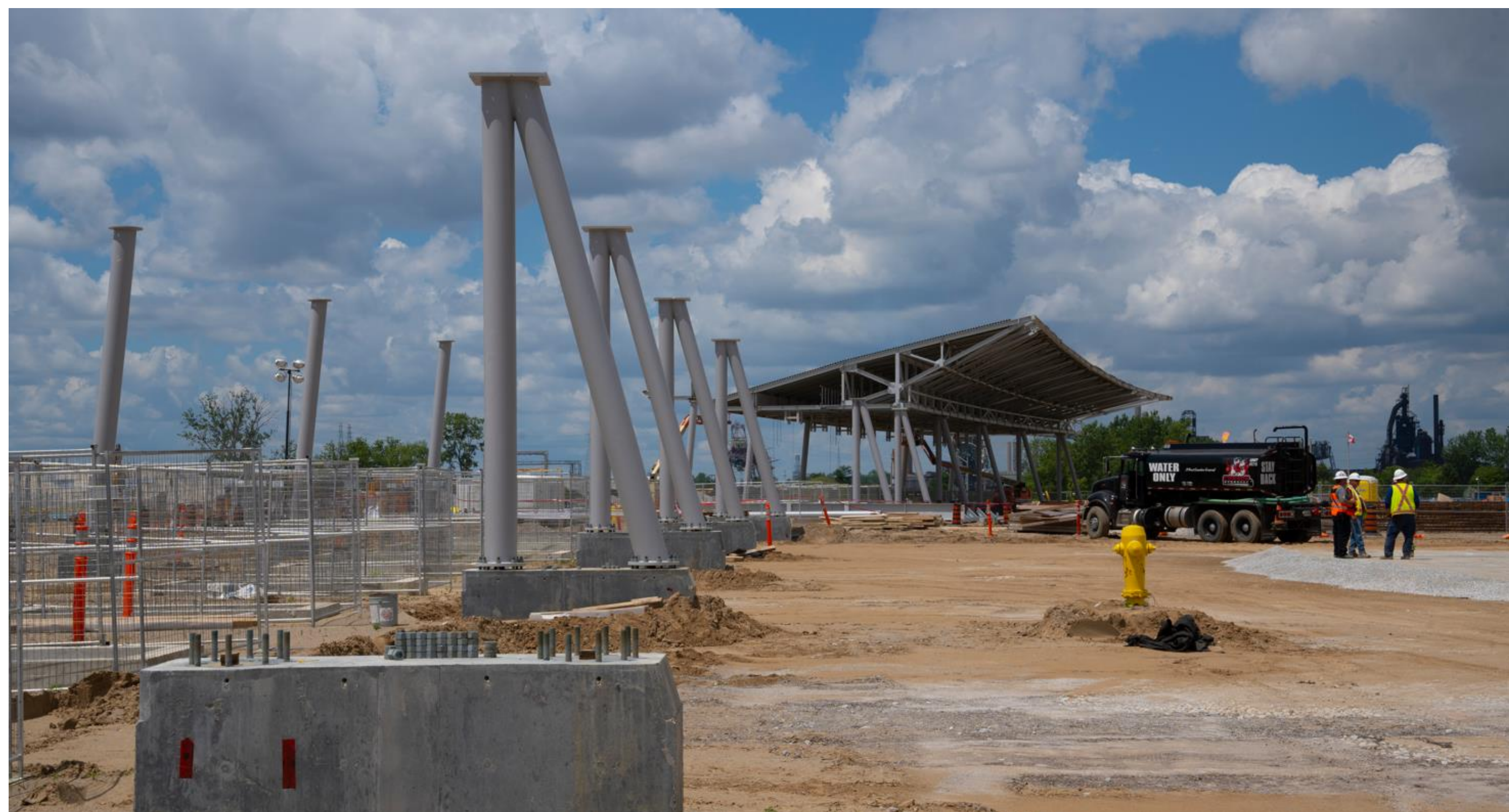
Canadian Port of Entry primary inspection lane canopy
