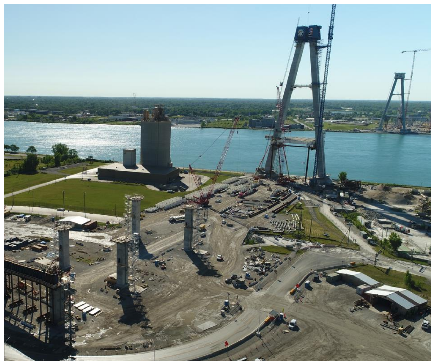
US bridge site: tower and side span work
