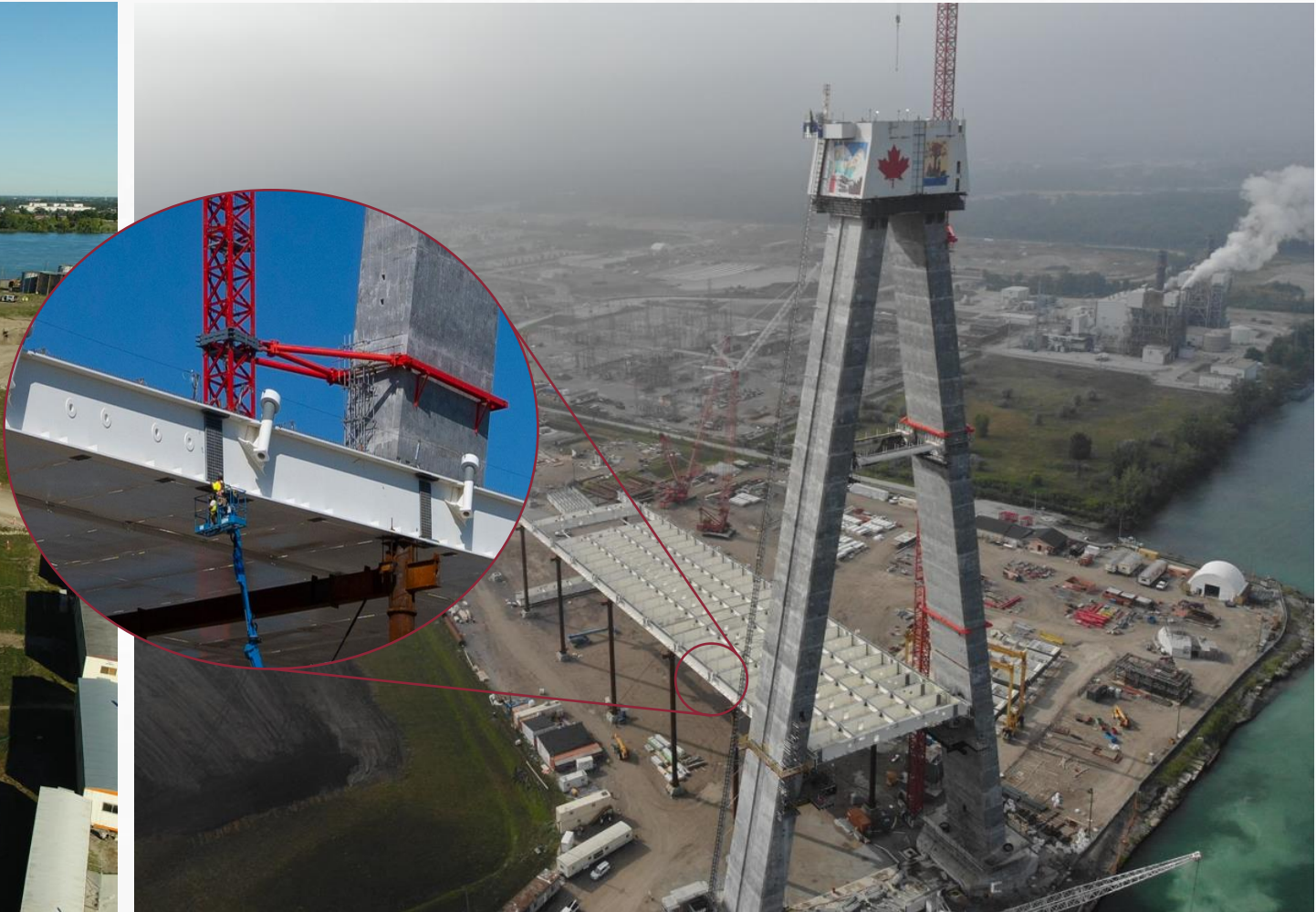
Canadian bridge deck construction
