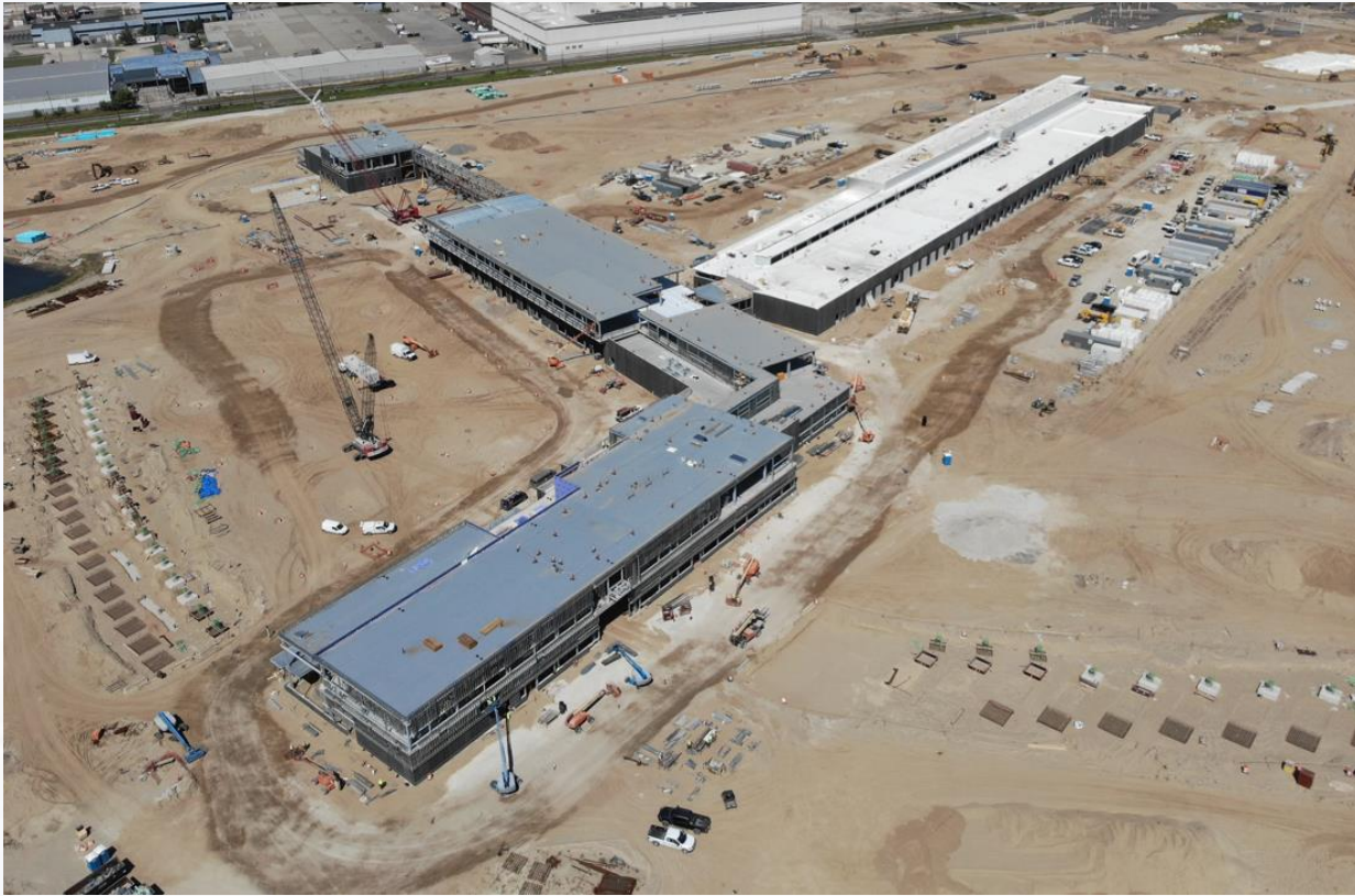
US POE building construction
