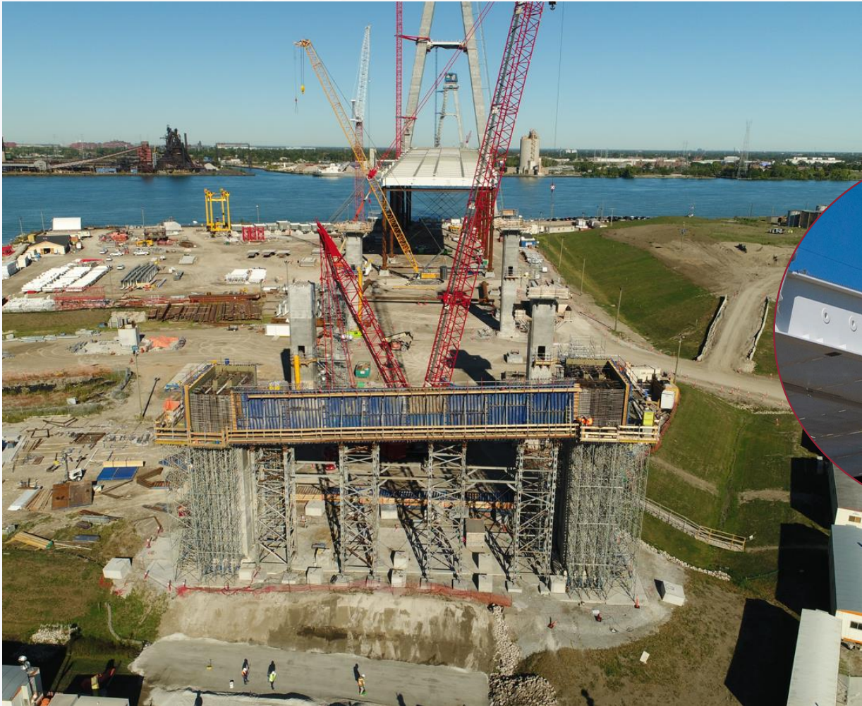
Canadian bridge site back span and bridge towers
