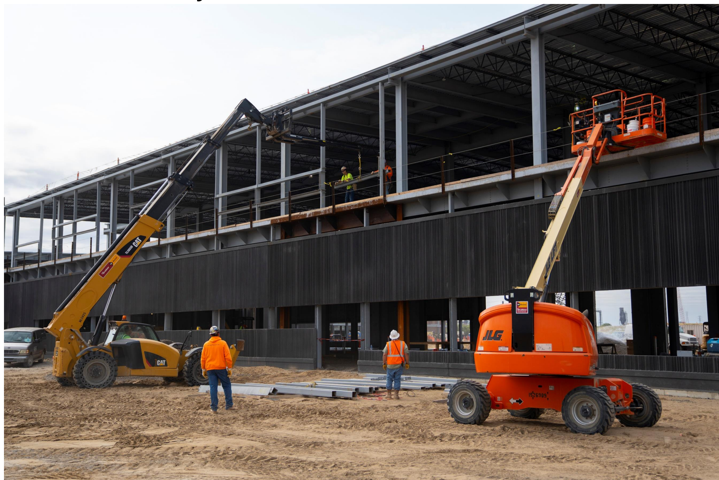
US POE facility construction
