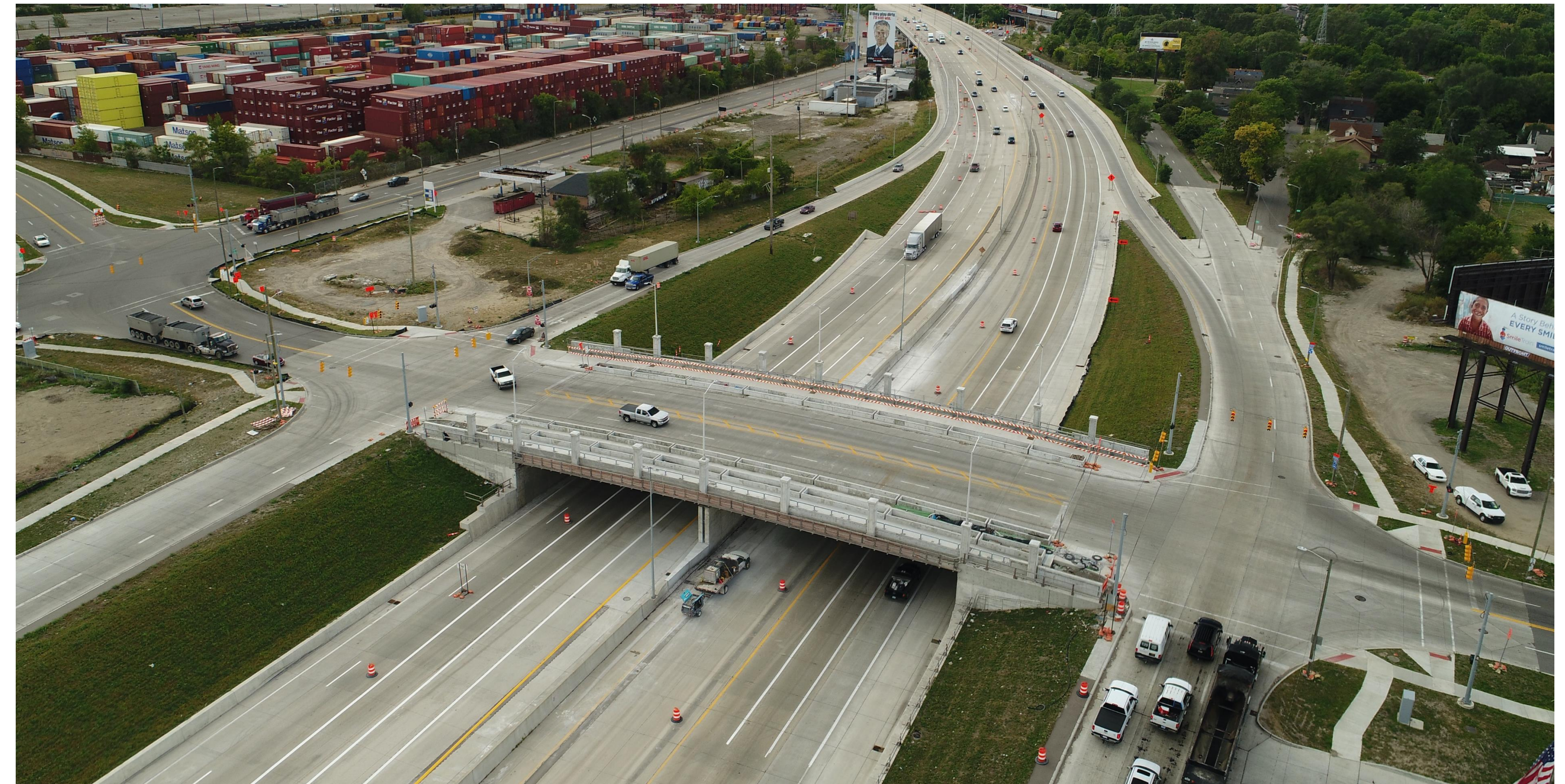
Springwells Street road bridge
