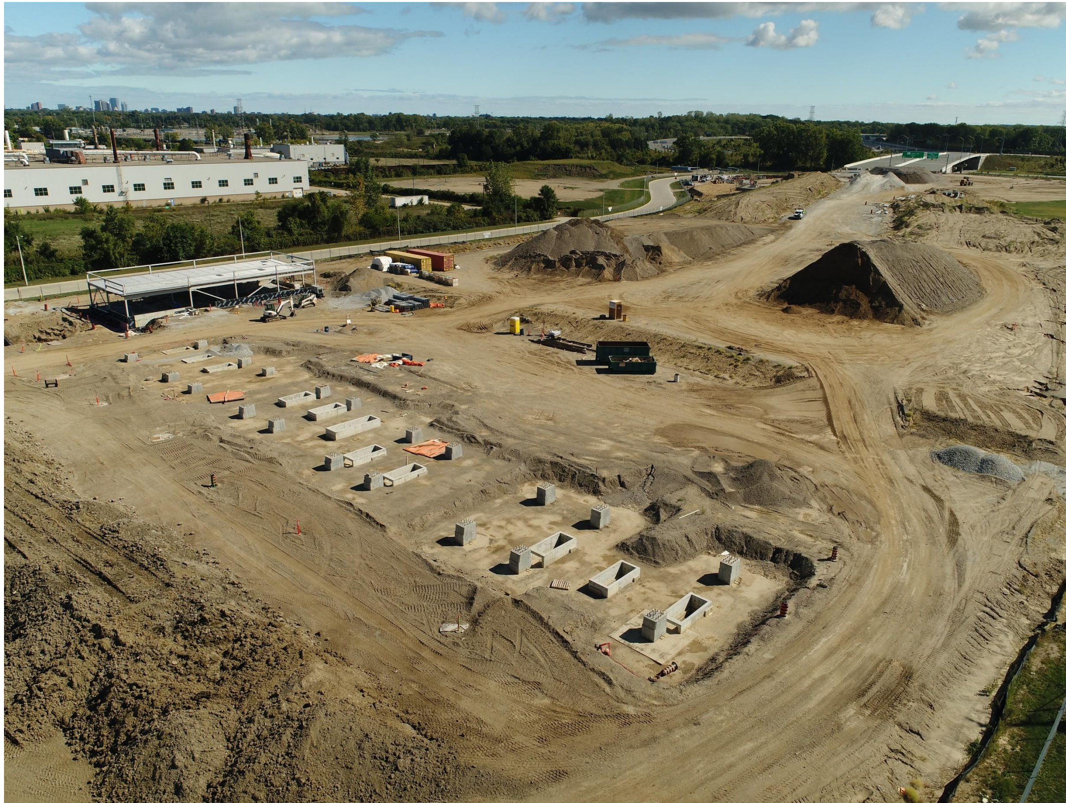
Canadian Port of Entry toll booths and east gateway construction
