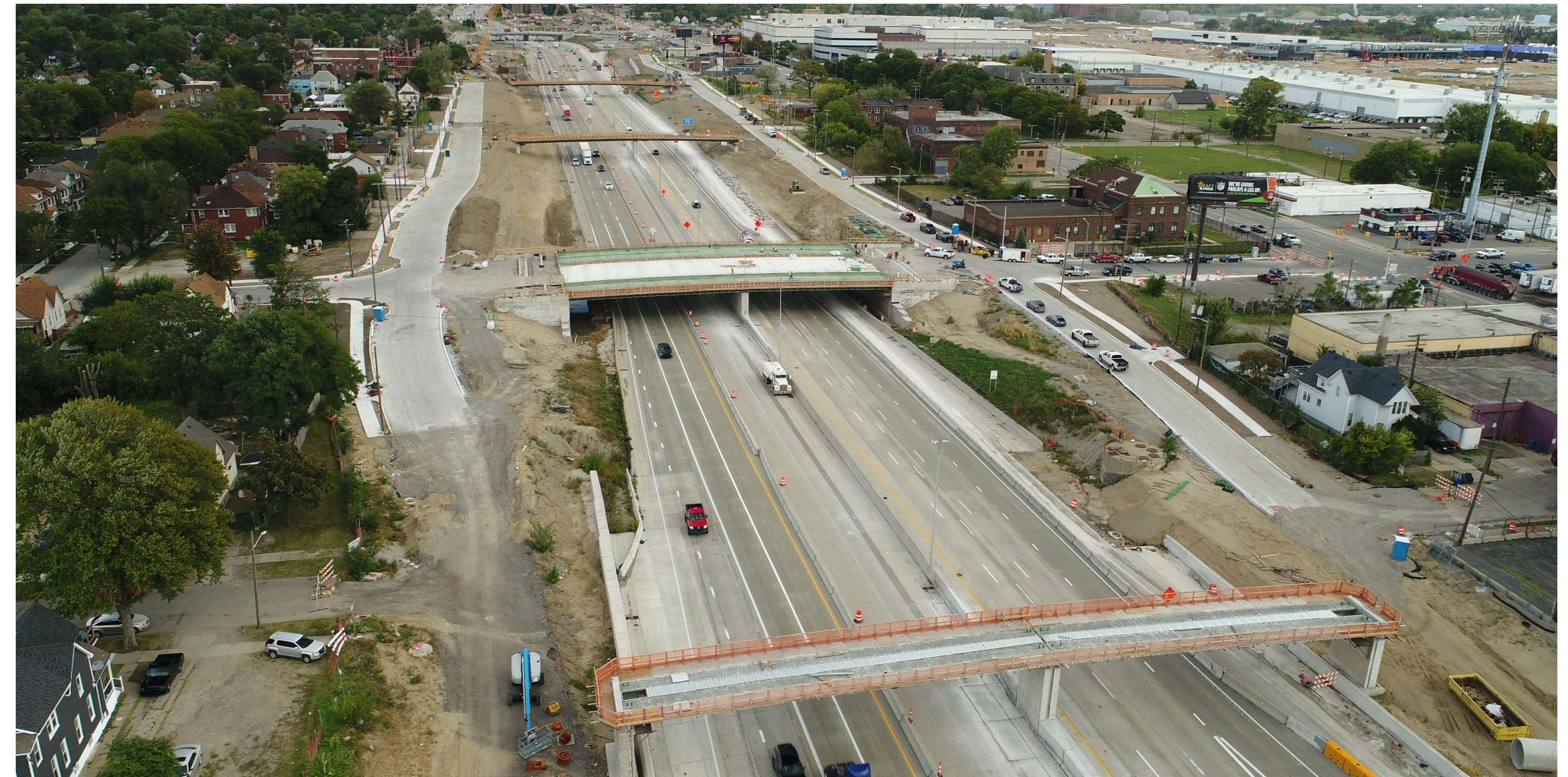
I-75 road and pedestrian bridge construction
