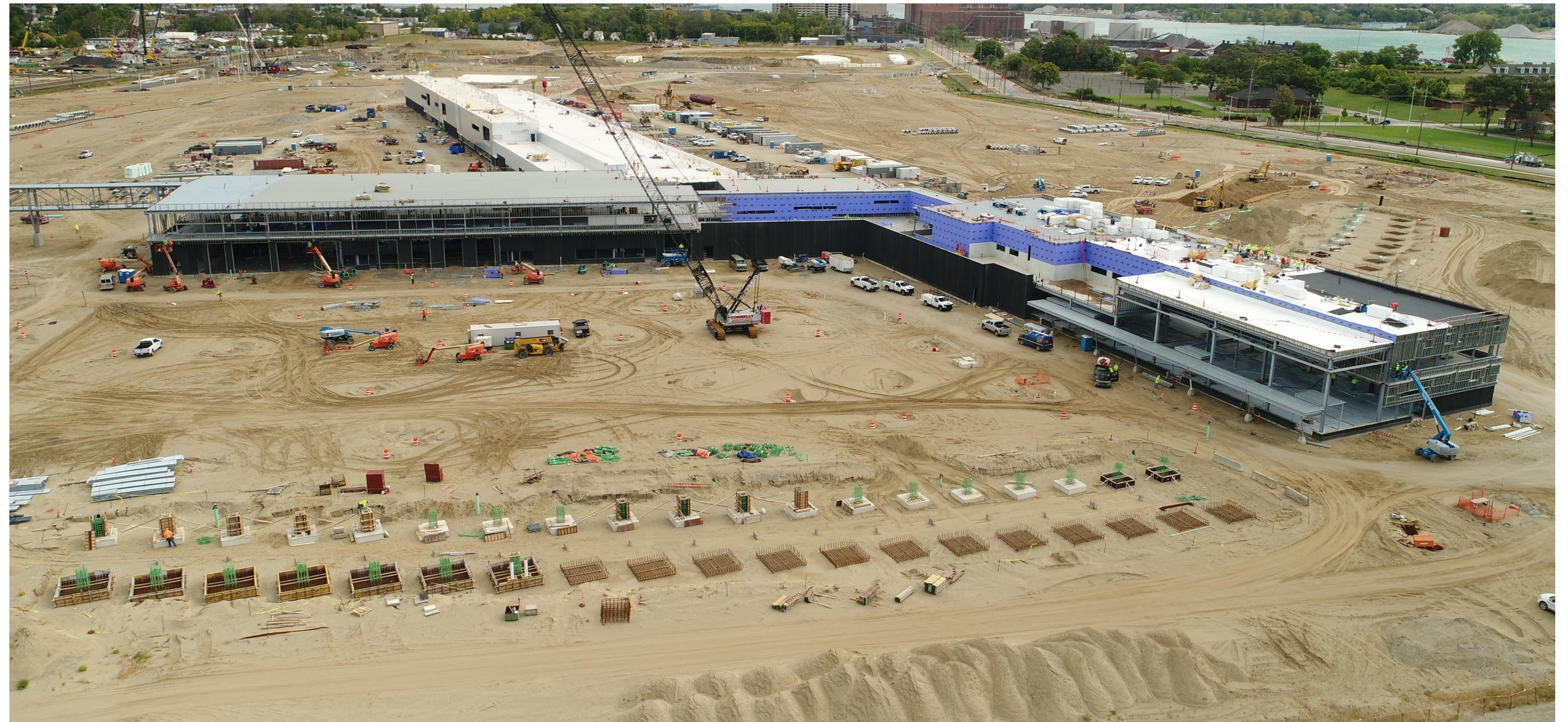
US POE facility construction and inspection lane foundation work
