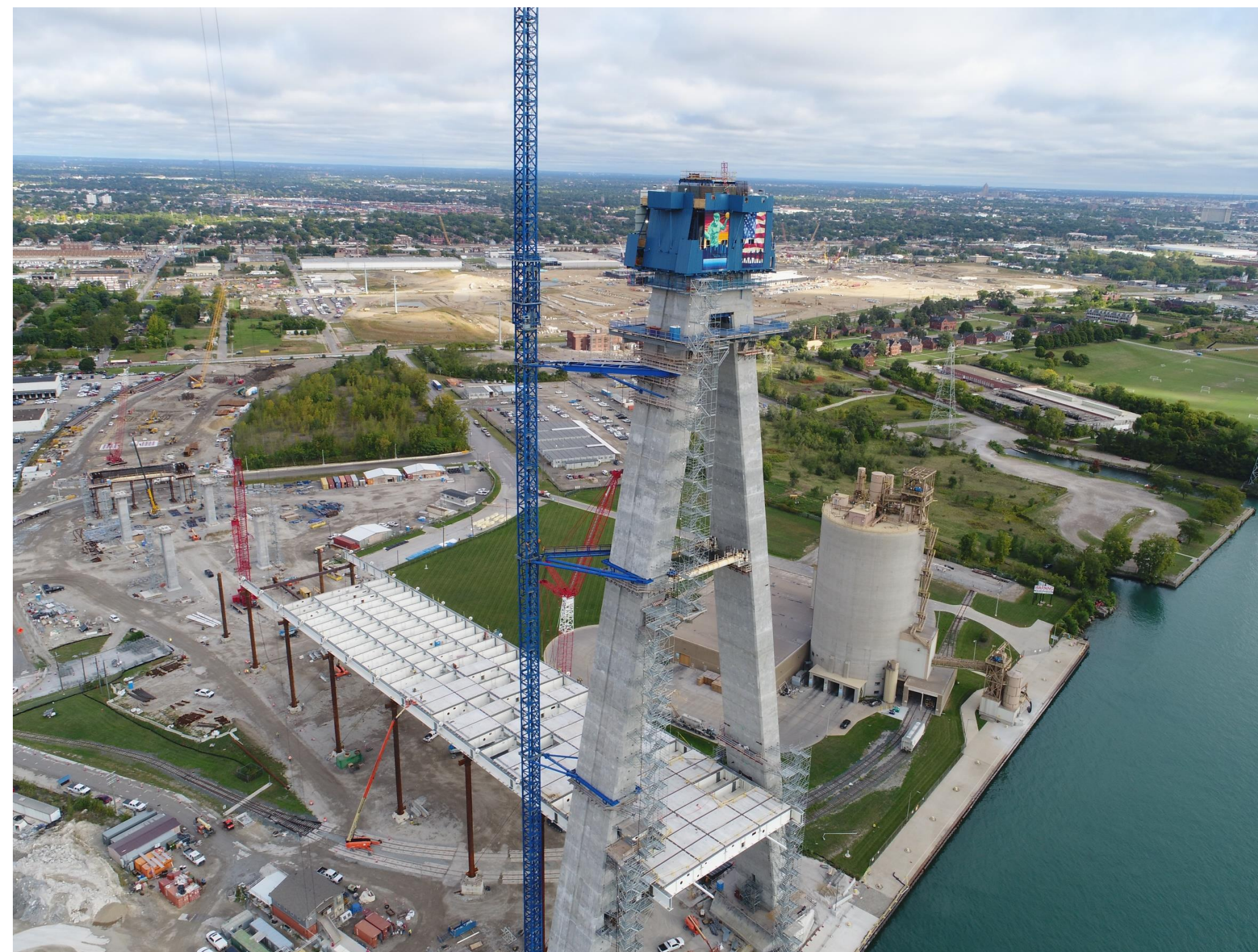
US bridge site: (left) bridge deck and side span work, (right) bridge tower work.
