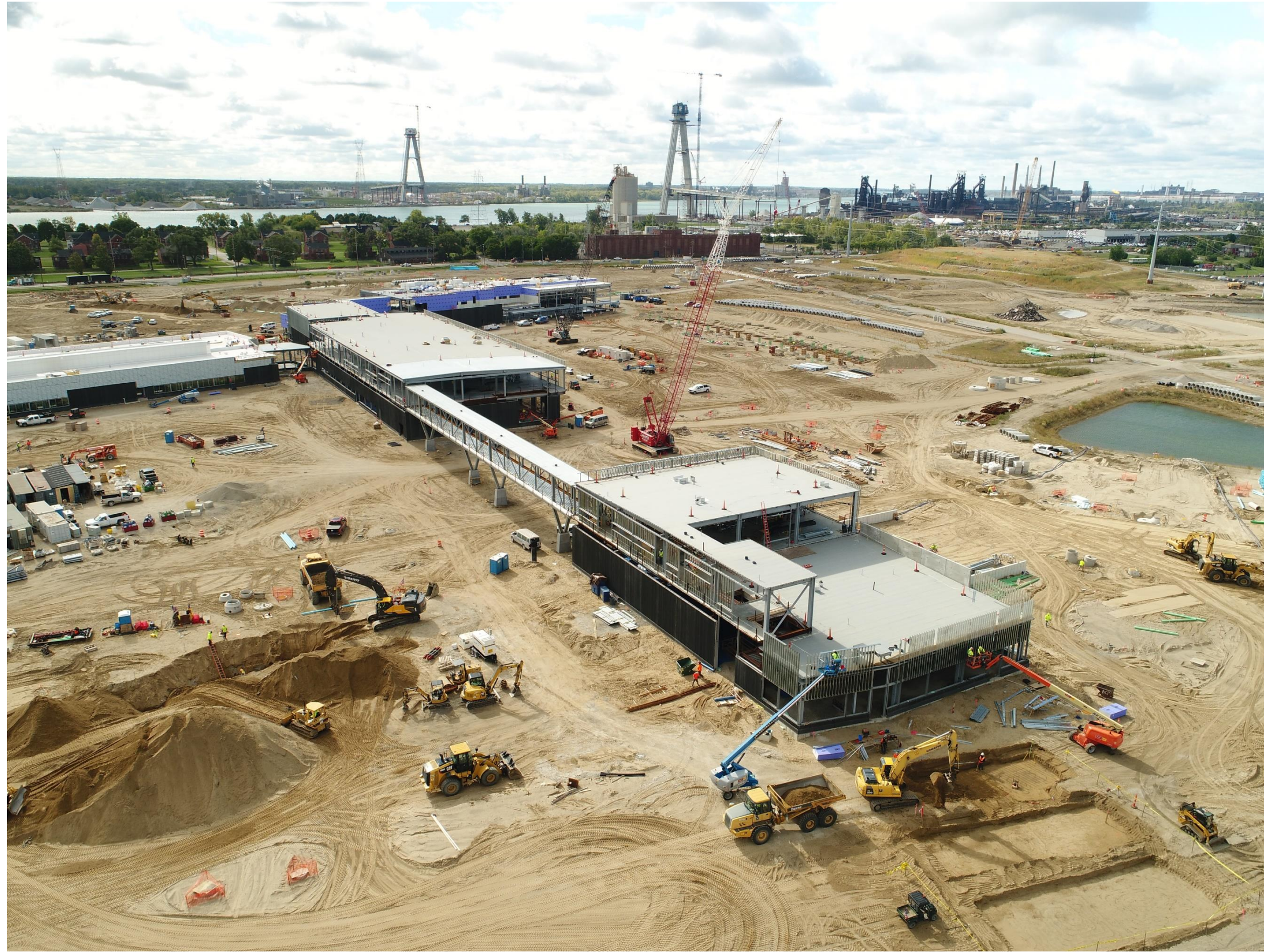
US POE facility construction
