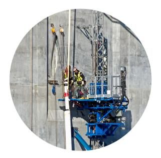
**Step 4:** Workers stationed on the mast climber take the reference strand and feed it into the anchor box inside the tower. Another crew of workers stationed inside the anchor box takes the reference strand, anchors it, and secures it with a steel wedge.
