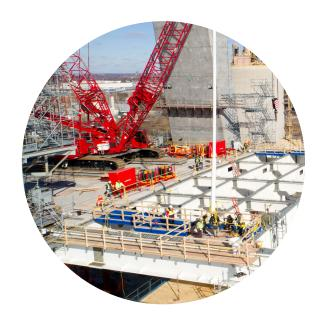
**Step 6:** Once both ends of the reference strands are secured, the process is repeated for the rest of the metal strands in the pipe. Each stay cable has between 38 and 122 strands inside.
