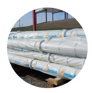
**Step 2:** Once welded, the first strand – referred to as the "reference strand" – is inserted into the pipe.
