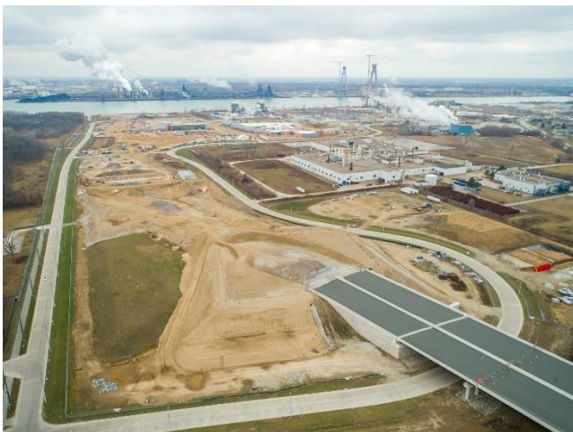
Canadian Port of Entry construction
