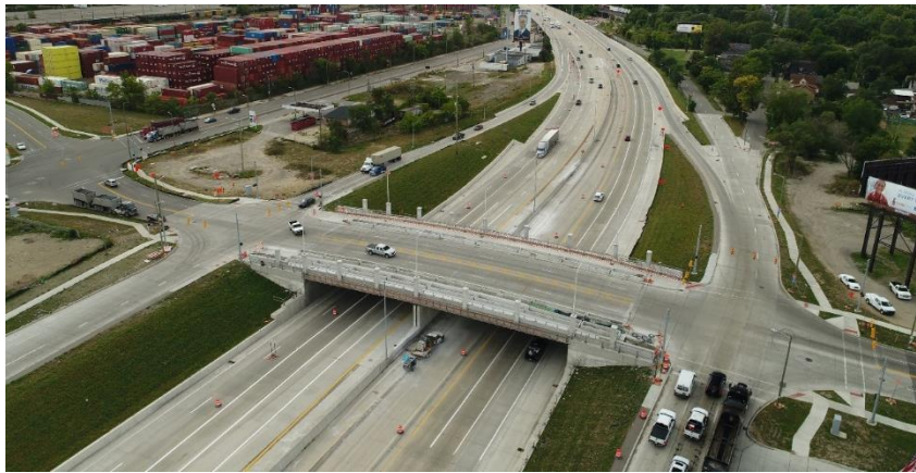
Springwells Street road bridge
