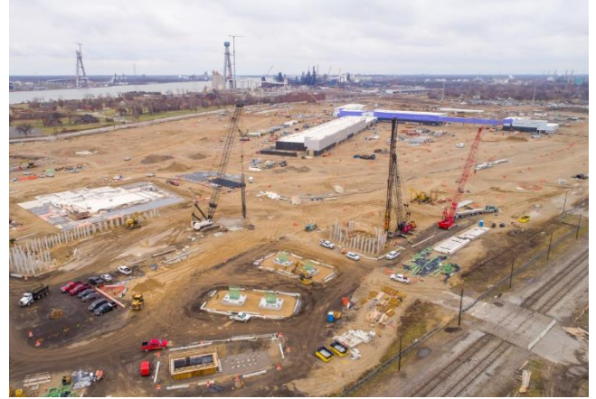
US Port of Entry construction
