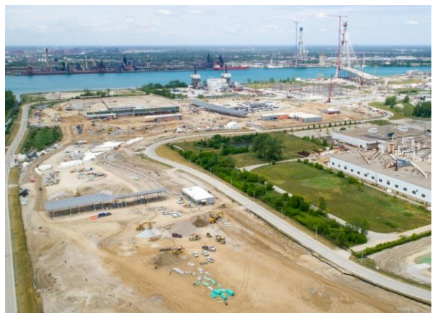
Canadian Port of Entry construction.
