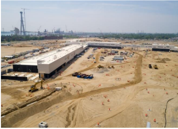
US Port of Entry construction.
