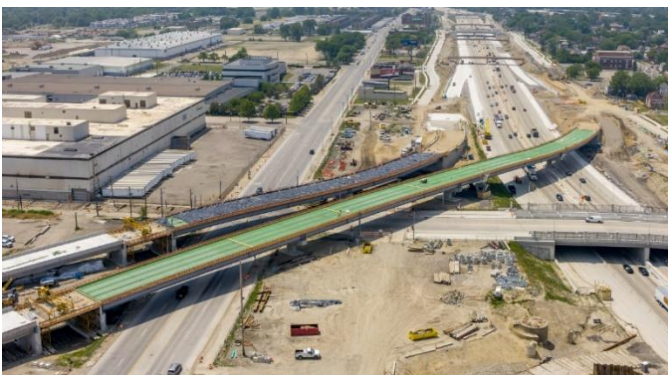
I-75 to US POE ramp construction.
