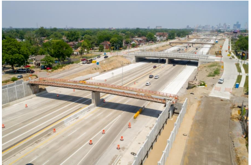
Road and pedestrian bridge construction
