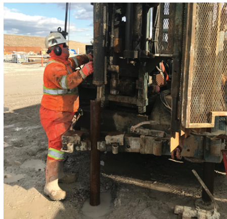
A drilling rig set up to extract a core sample
