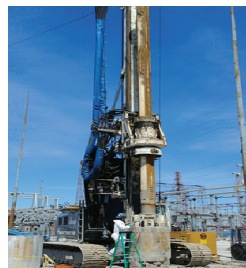
The complete drill rig setup
