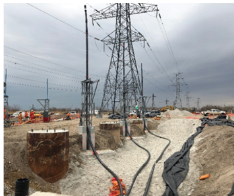
The cabling being connected to a transmission tower
