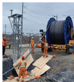
Cable being pulled from the spool
