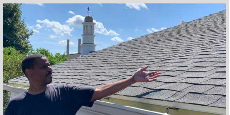
Forest Hudson shows off the gymnasium's new gabled roof
